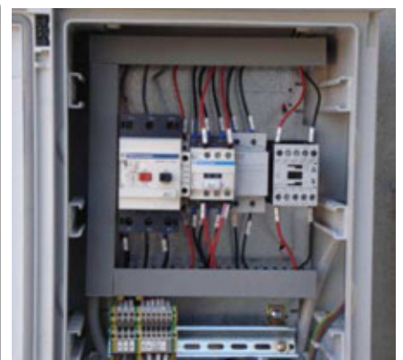
Circuit inside the electrical panel
