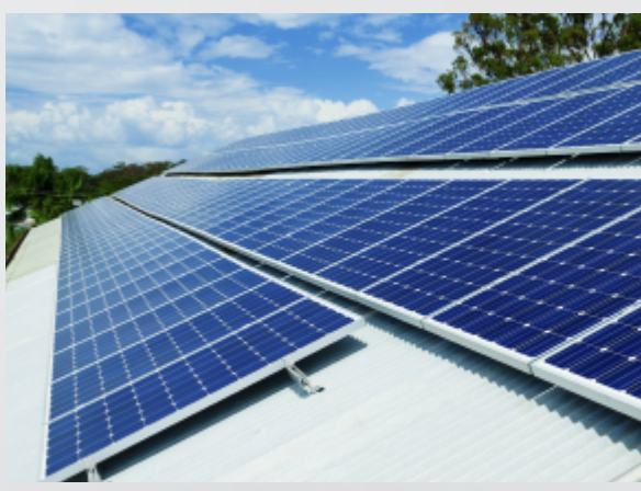
Energy Storage System (ESS)
