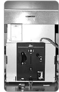
VCB (Vacuum circuit breaker)
