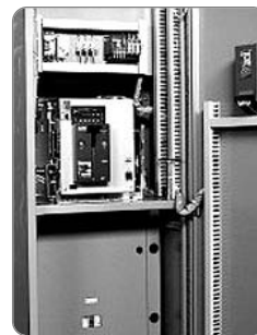
ACB & MCCB (Mold cased circuit breaker)
