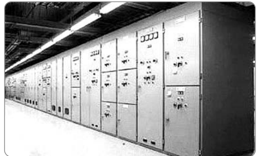
LVS (Low Voltage Switchgear)
