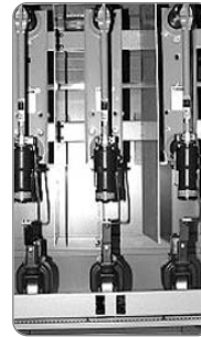
PT (Voltage transformer) & PF (Power Fuse)
