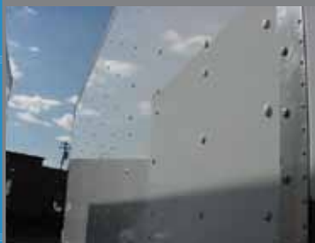
Previous process. Note the through-bolts.
