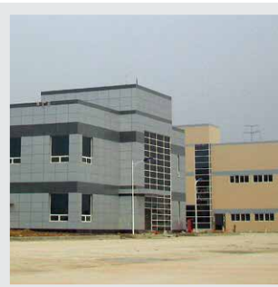
Wuxi Plant (China)
